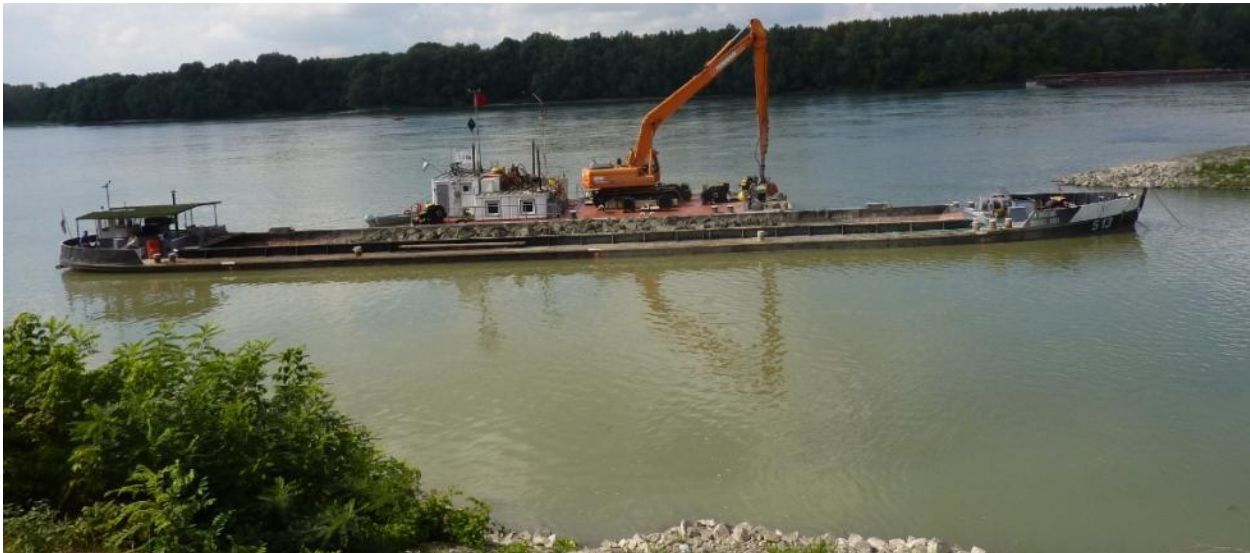
Figure 30: Spoon dredger with self-emptying barge on the Danube
